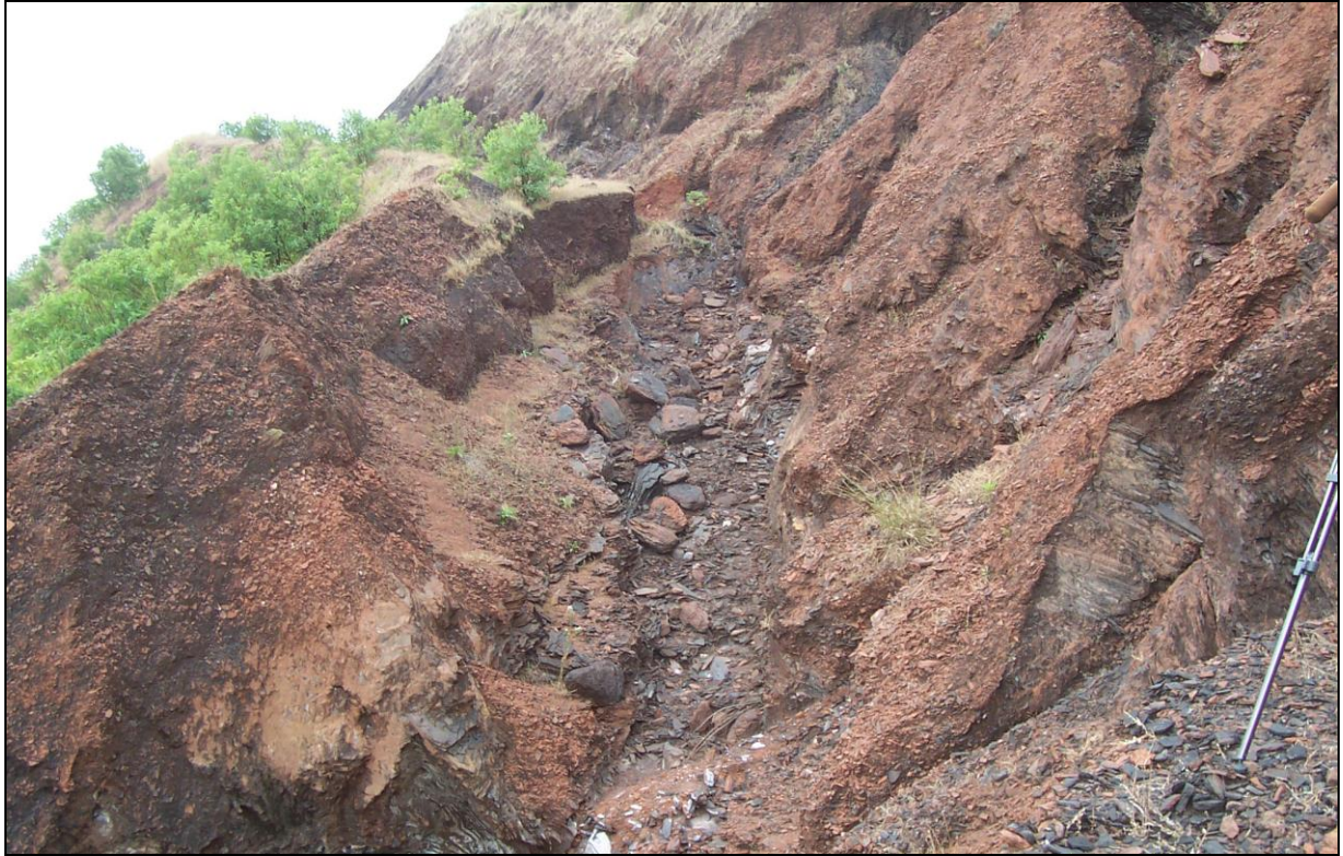
Photo 3: The Depletion zone of the Landslide caused due to mining activity at Ambargudda area.
